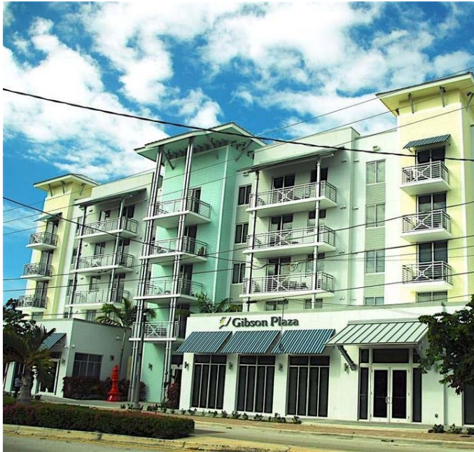
Gibson Plaza, a new mixed-income senior housing development in west Coconut Grove. Pinnacle Housing Group
