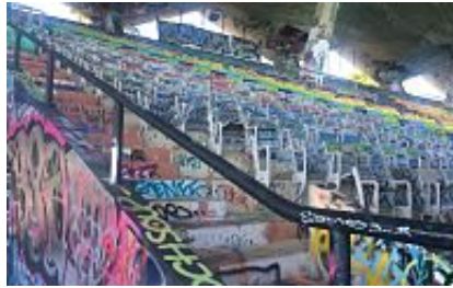
Commissioners approve $16M in upgrades to Miami Marine Stadium
